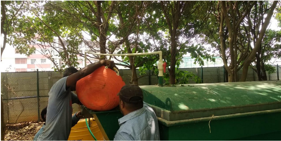
Feeding into Bio-Digester
