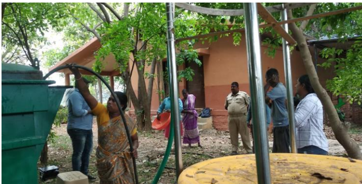
Connecting biodigester to gas collection tank
